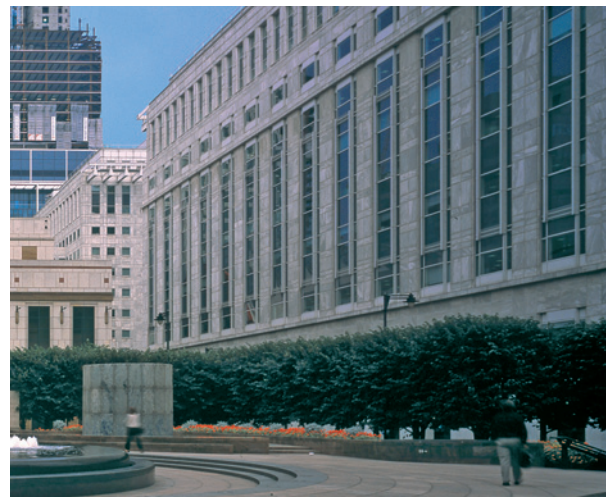
Building façades and perimeters
